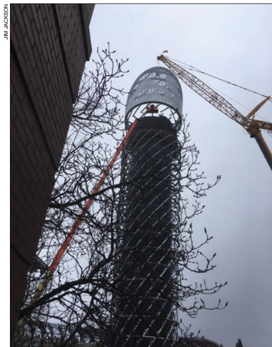
As construction continues on the new Hayward Field, the signature tower got its cap on February 1.
